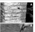
Push out the 2 screw covers using a flat screwdriver at the back of the external caller unit.
